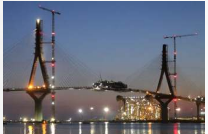
Construction of the Puente de la Pepa bridge in Cadiz, Spain
