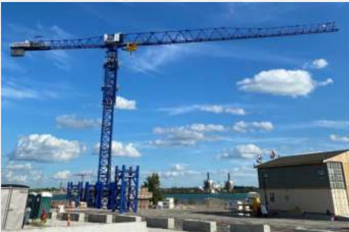
Gordie Howe International Bridge between the USA and Canada
