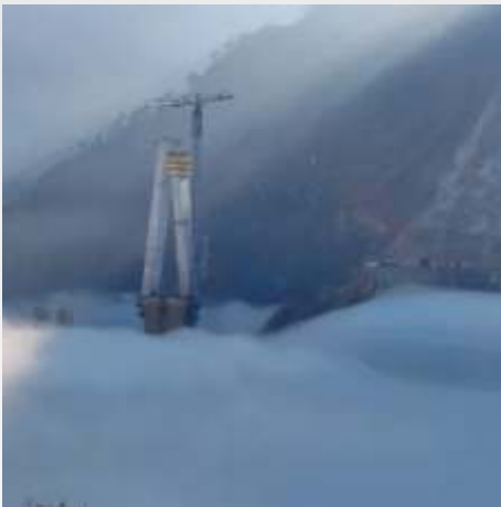
Anji Khad Bridge in India
