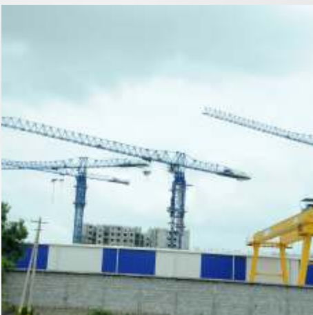
Shapoorji Pallonji. Tata Housing Project, Bangalore
