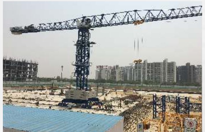
KEF (Kattera India), Lulu Mall Project, Lucknow
